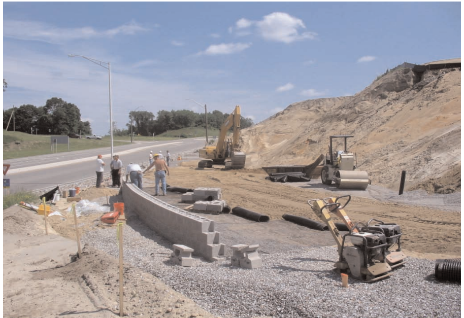
First course of block at lowest elevation.
