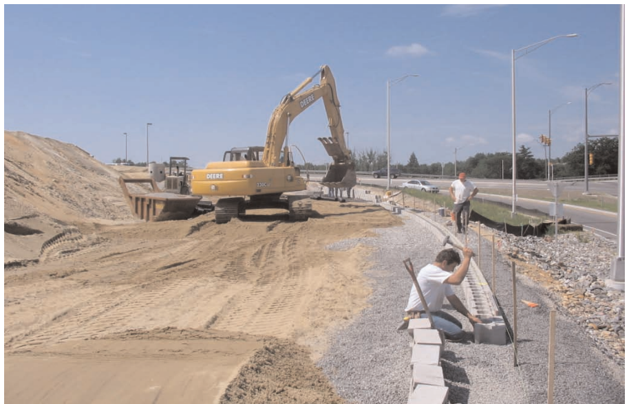
Placing blocks on leveling pad, forming radius
