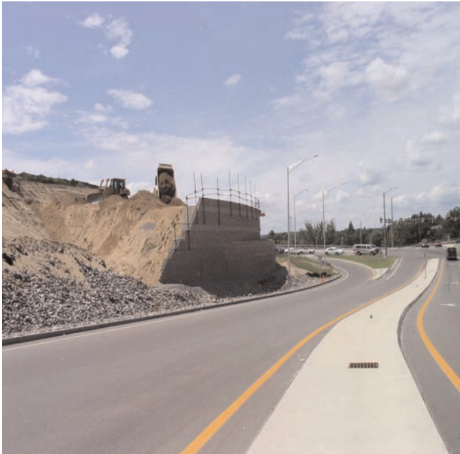
Tiers coming together at the end of the wall.
