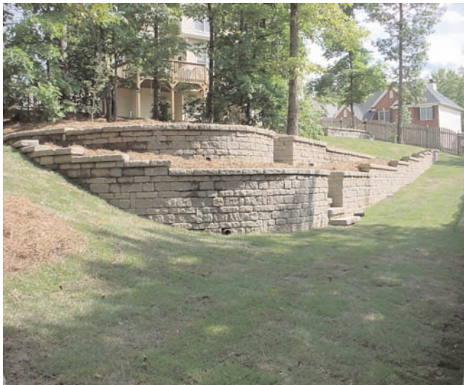
Final backyard: Lower tiered retaining walls; middle retaining wall, above-right.
