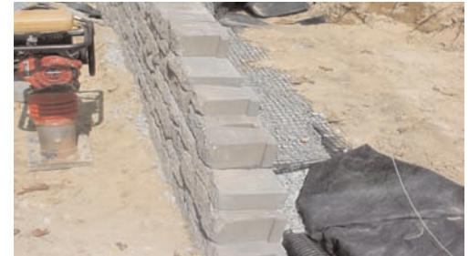
Lower retaining wall construction: Alternate perspective.
