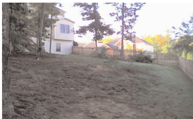
Initial backyard conditions: Lower retaining wall area.
