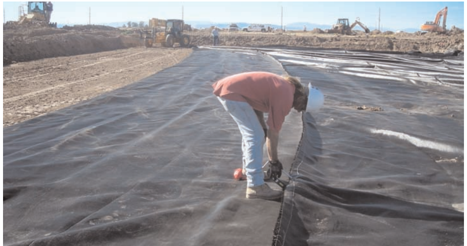
Mirafi® HP570 pulled in place using C-clamps at field sewn joints.
