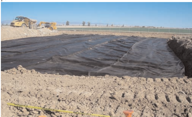
Mirafi® HP570 sewn panels placed on the subgrade.
