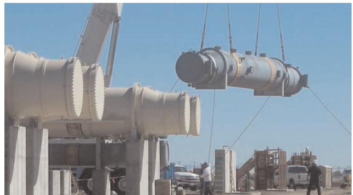
Heavy geothermal power equipment placed on stabilized Mirafi® HP570 platform.
