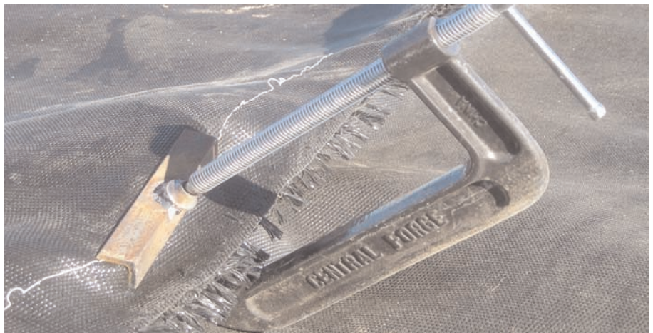
C-clamp at field sewn joint.
