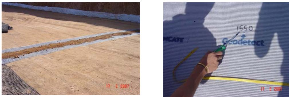
Figure 6. Placement of the 'intelligent' geosynthetic strip.
