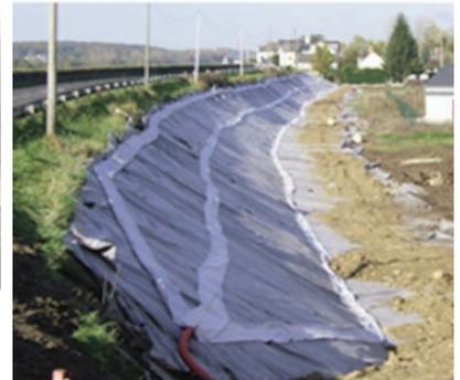
Three TenCate GeoDetect® S-BR strips on the Loire river levee.
