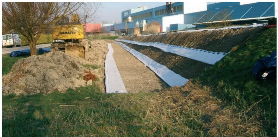
The GeoDetect® S-BR strips on the Marne to Rhine canal.
