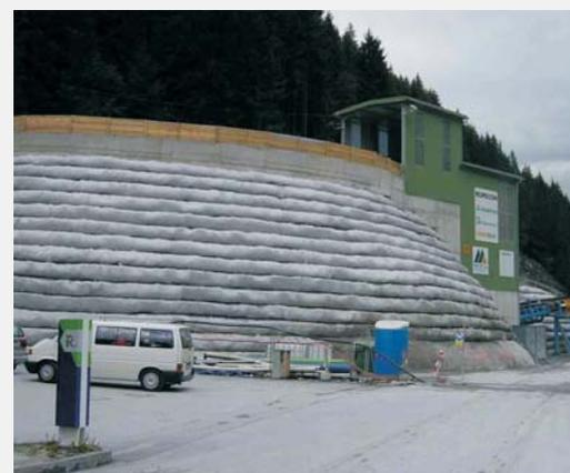
(e) Polyslope T without facing (temporary structure)
