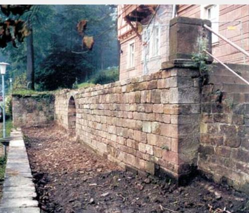
(c) Polyslope T with dry masonry facing
