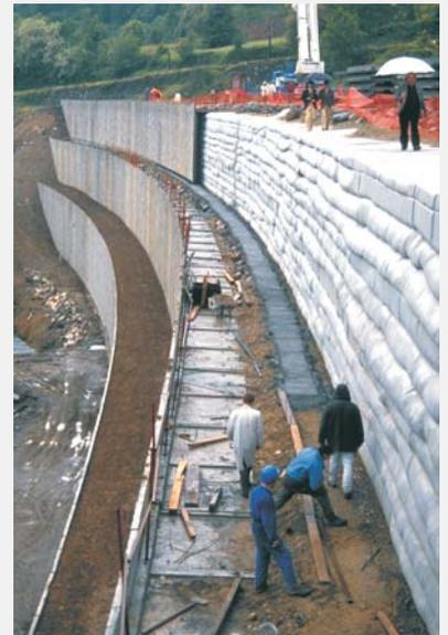
(a) Polyslope T with precast concrete facing
