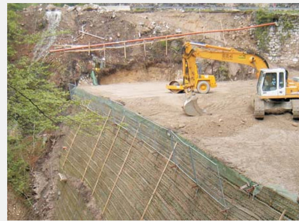
Quick, easy and economical installation as well as optimum conditions for plant growth are the main characters of the Polyslope S System (top: construction phase, below: condition after one year).
