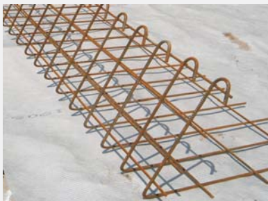
Prefabricated steel meshes acting as lost formwork elements
