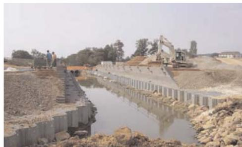
Figure 6: Embedding the TenCate GeoDetect® strips and instrumentation cables into the fill material.
