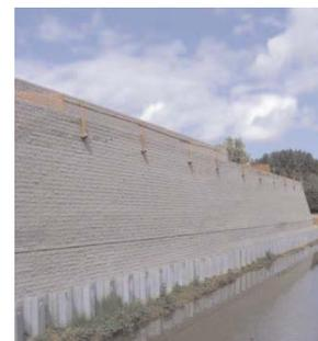
Figure 1: View of finished wall bridge abutment walls with “Leromur” concrete block facing.
