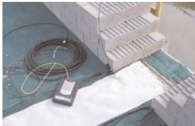
Figure 3: The elements of the TenCate GeoDetect® equipped wall system: (1) Leromur blocks (2) reinforcing geosynthetics (3) GeoDetect® strip (4) outdoor cable (5) hand-held measuring device.
