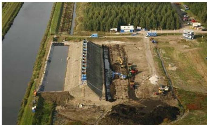
Figure 4: Aerial view of the IJkdijk experimental dike during the macro-stability experiment, the upstream basin on the left filled with water, loading containers on top, and the trench digged out 2 m from the dike toe.
