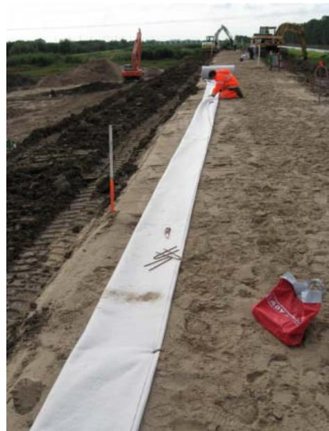
Figure 3: Installation of one GeoDetect® S-BR sensor strip in the IJkdijk macro-stability dike.
