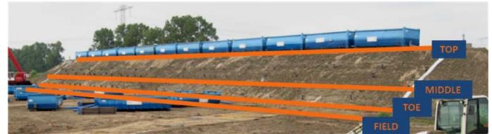
Figure 5: Placement of the 4 GeoDetect® sensor strips along the IJkdijk macro-stability dike, at the crest (TOP), at the middle of the slope (MIDDLE), at the dike downstream toe (TOE), and 2 m from the downstream dike toe (FIELD).
