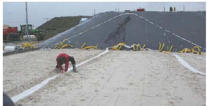
Figure 10. Installation of the GeoDetect® sensor strips embedding both strain and temperature fiber optics 10 cm into the sand layer before construction of the dike.
