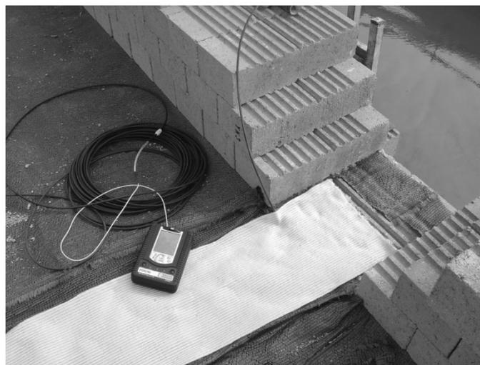
**Figure 3. The GeoDetect<sup>®</sup> strip No. 2 installed**
