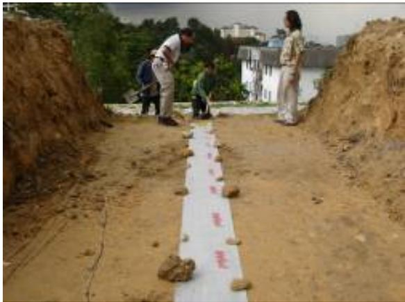
Fig.7 Trench excavated at the top of slope for placement of the geosynthetic to monitor movements of existing slope
