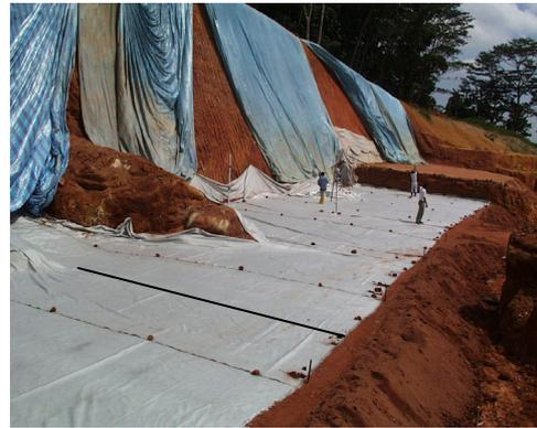
Fig. 6(a) 'Intelligent' geosynthetic placed in the structure as part of the soil reinforcement system
