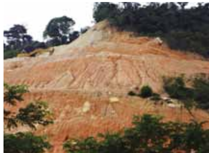
Bare slopes erode without protection
