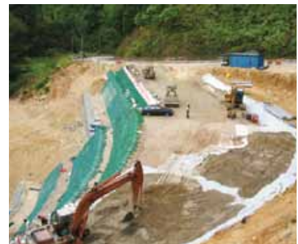
Figure 3: Reinforcing slope with Polyfelt® PEC.
