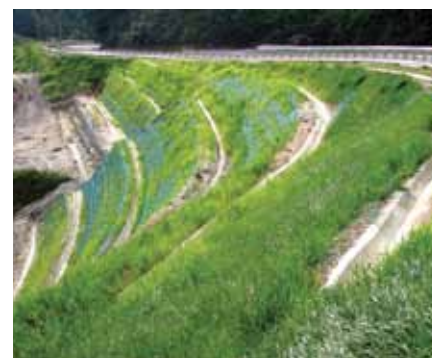
Figure 4: Vegetated slope after completion.
