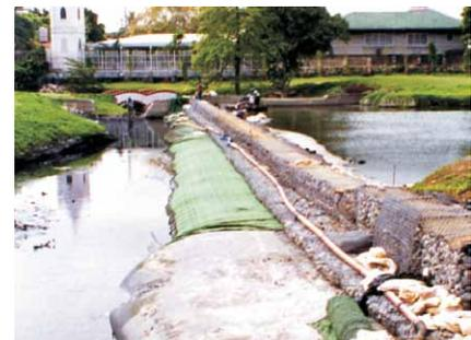
*Installation of the Gabion above the Geotube<sup>Æ</sup> engineered tubes*
