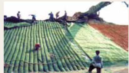
Geotube® Sand Filled Mattress being filled hydraulically with sand.
