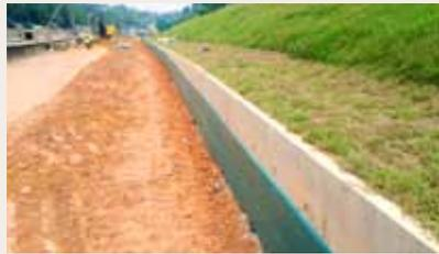
Mirafi® Silt Fence installed to prevent silt from spilling into the drain.
