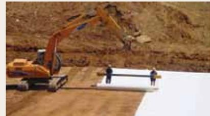
Laying Polyfelt® Enviromat GCL using crane.
