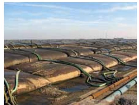
**Three layers of Geotube<sup>®</sup> containers on the dewatering platform**
