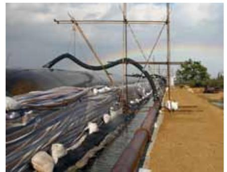
**Filling Geotube® containers with contaminated sediments**
