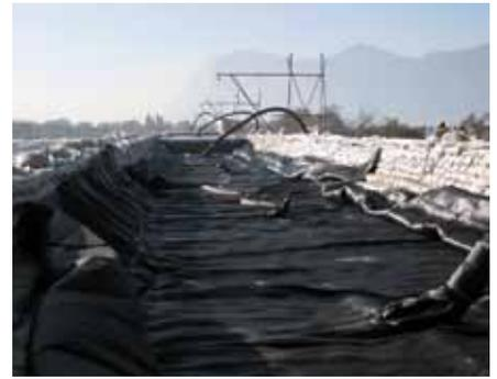
**Installing Geotube® containers inside the geobag buttress walls**
