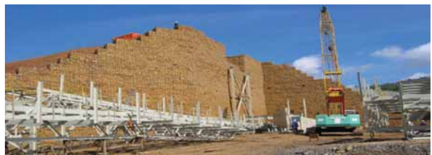
Figure 4: Typical sample of a completed Polyfelt PEC reinforced gabion dump wall
