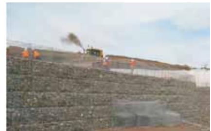
Figure 3: Construction of wall in progress
