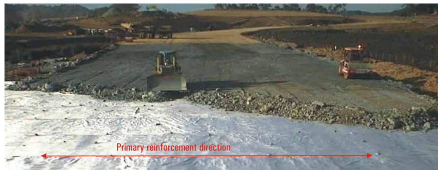
Installation of the high tenacity Mirafi® PET geotextile
