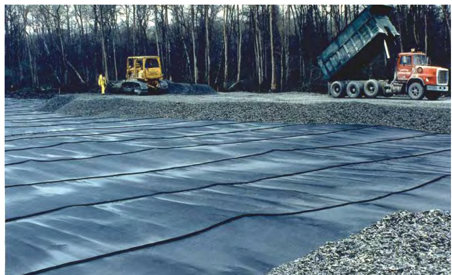
Installation of road base fill over the Mirafi® HP geotextiles
