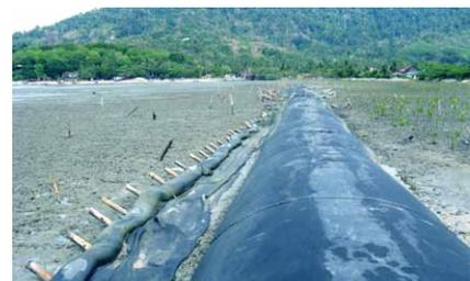
Geotube® containment unit was installed on top of bamboo mattress.
