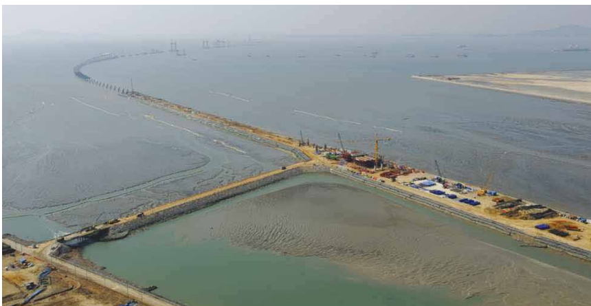
Overview of the Geotube® working platform
