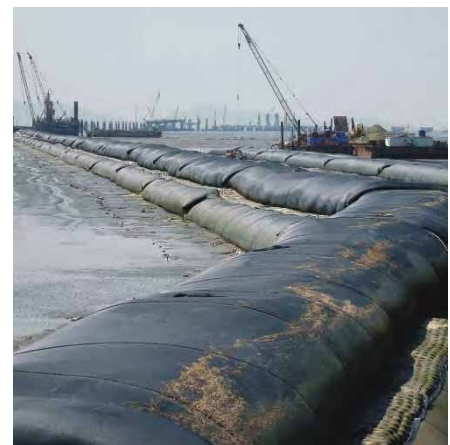
Geotube® GT1000 along the edge of the reclaimed platform
