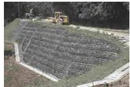
Slope repair works in progress
