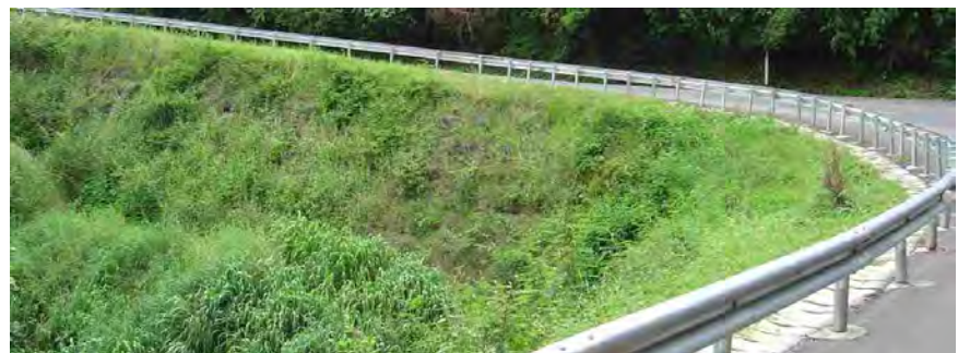
The completed Miragrid GX reinforced slope with vegetation fully established
