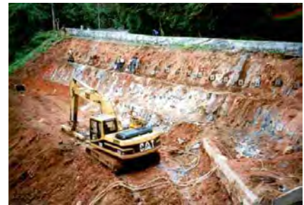
Soil nailing and slope base preparation
