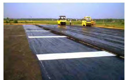
Figure 3: Overlaying of 50mm thick ACWC on PGM-G 50/50.
