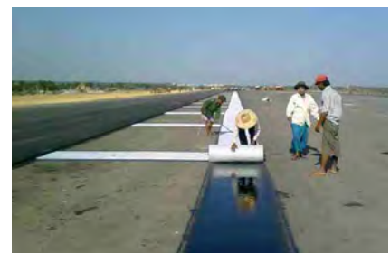
Figure 2: Installation of PGM-G on longitudinal construction joints.
