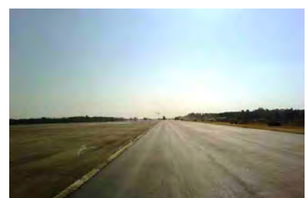
Figure 4: Completed runway open for air traffic.
