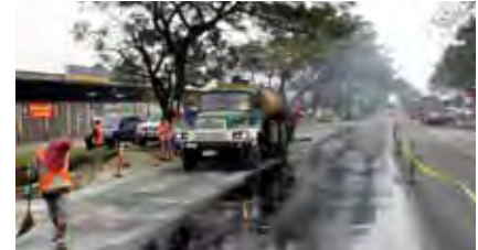
Spraying of tack coat by using a bitumen tanker.
