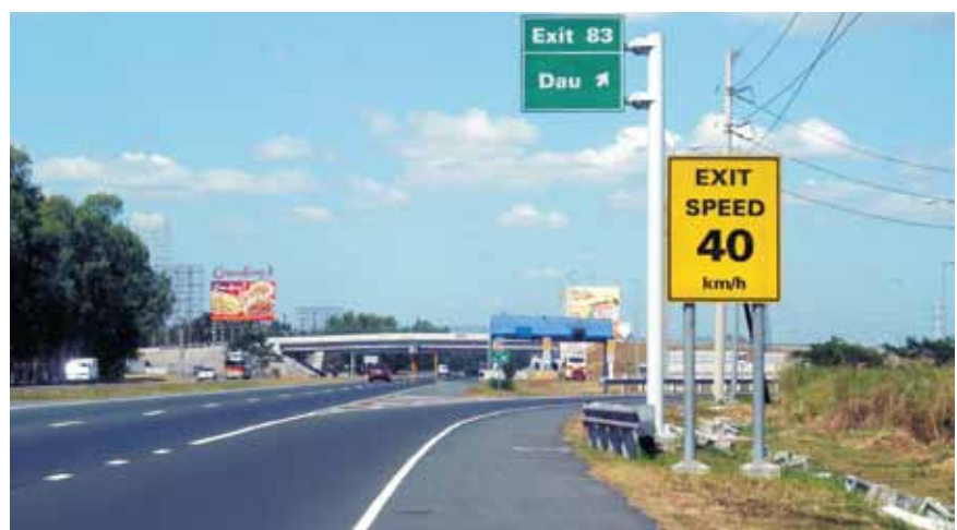
Completed road section opened for traffic.
