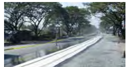
Installed Polyfelt® PGM14 paving fabric along the expressway.
