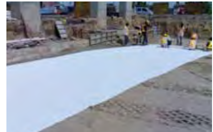
Installation of Polyfelt® WX300/50 as basal reinforcement.
