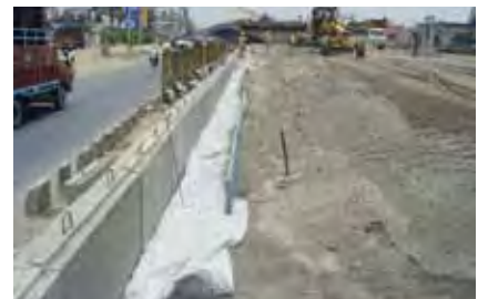
Polyfelt® TS filter behind the concrete fascia with Miragrid® GX reinforcement.
