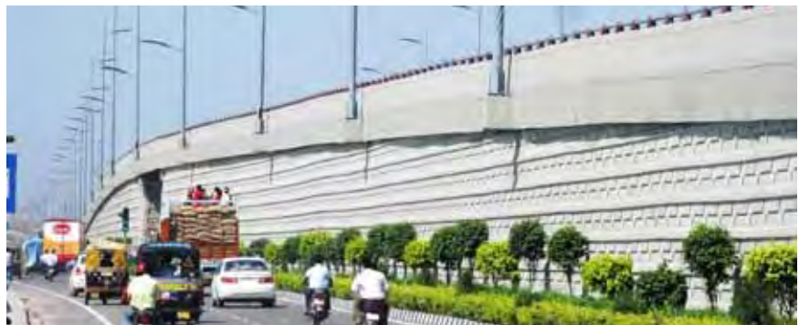
Completed reinforced soil wall for bridge approaches.
