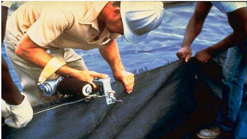
Two types of sewing equipment are most commonly used: a) a single needle, hand-held sewing machine, and b) double needle stitch sewing machine which is typically table-mounted. Figure 3 illustrates the field sewing of geotextiles using the hand-held machine.
