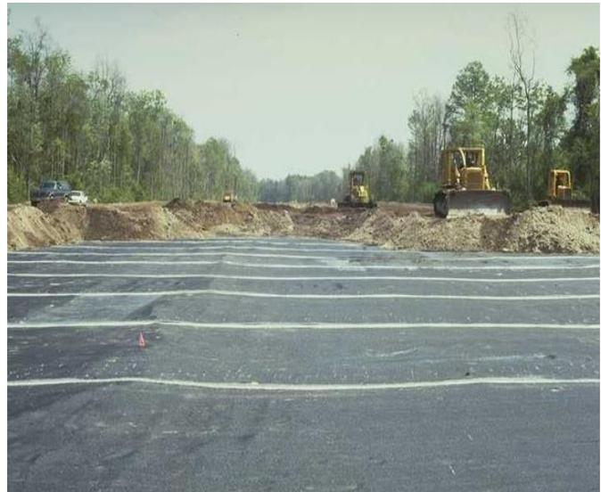
Figure 1. Seamed Geotextile Panel
