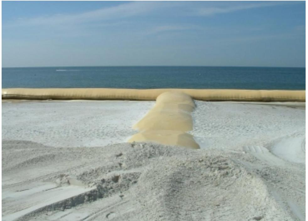
*T-groins using Geotube® containers were used at Upham Beach to control an ongoing beach erosion problem that had cost county officials more than \$10 million dollars. The T-groins began working immediately to stop erosion and allow the beach to renourish.*
