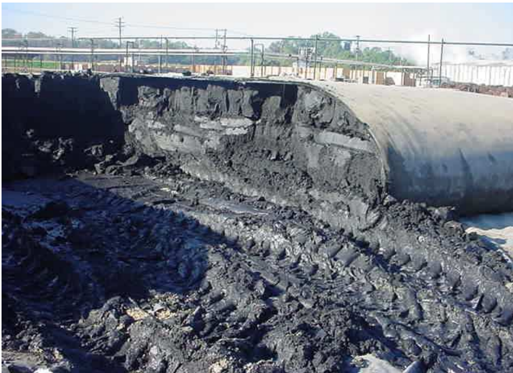
A Geotube® unit opened to show the dewatered ash inside. Often the material can be recovered and reused.
