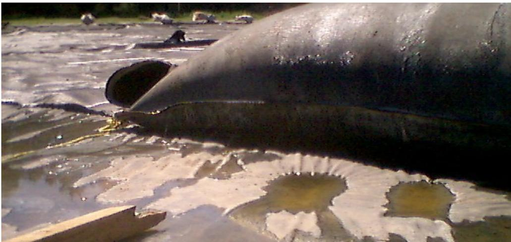
*Water drainage shows effectiveness of Geotube<sup>®</sup> units.*
