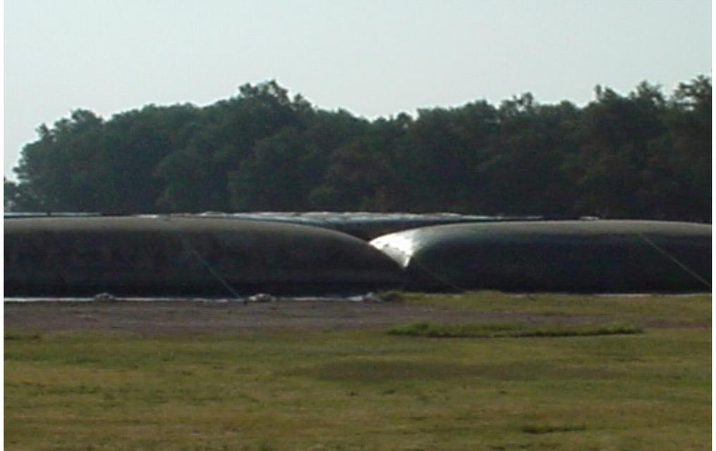
*Geotube® units installed on a baseball field next to the plant lagoons. Dewatering with Geotube® technology was extremely effective and was accomplished in much less time and with less expense than mechanical dewatering. If needed, more units could be stacked on top of these.*
