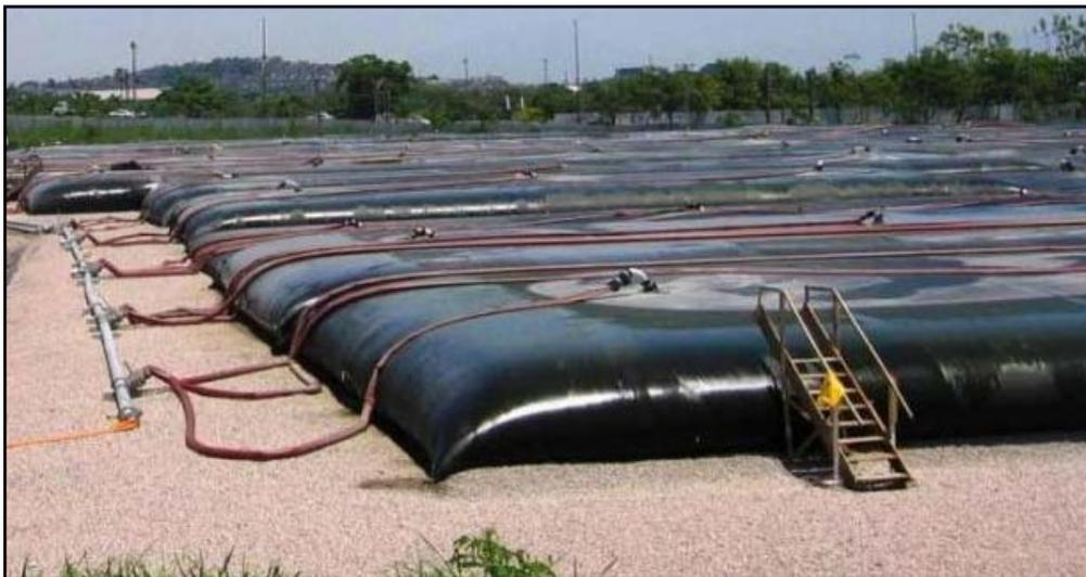
*Geotube<sup>®</sup> dewatering containers are supported by a Miragrid<sup>®</sup> 24XT base layer in the dewatering cell. As the project is completed, this area will be covered and developed into new green space.*
