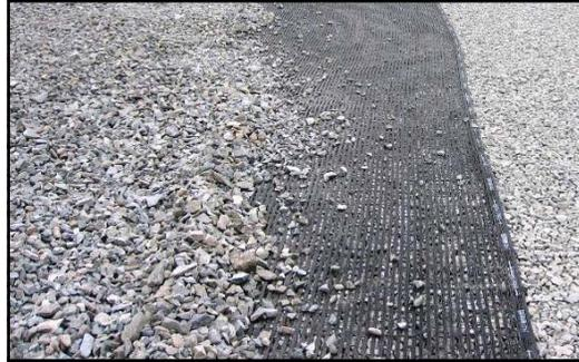
Miragrid® 24XT reinforcement was installed between two layers of base stone. Its simple installation took two weeks.
