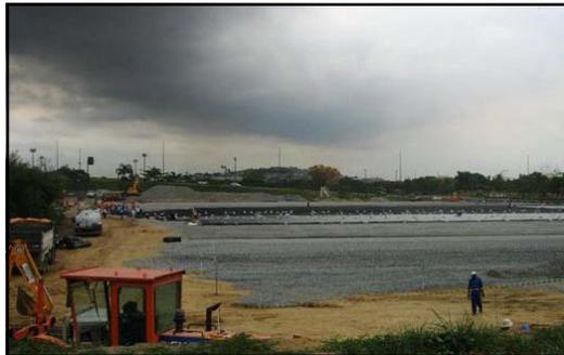
Construction of the dewatering cell utilized reinforcement layers of Mirafi® 1160N non-woven geotextile for safety.
