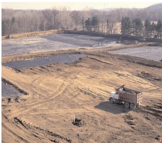
Mirafi® GC1000 was used to cap this sludge lagoon.
