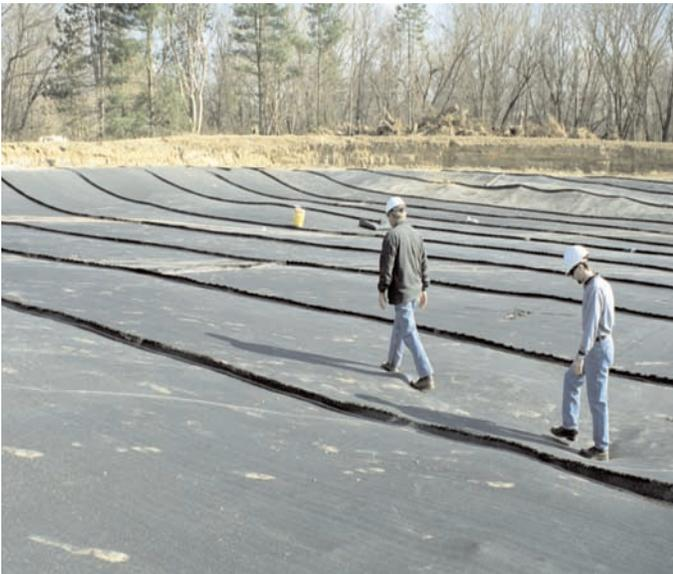
Three layers of Mirafi® GC1000 were placed on the east section of the lagoon. One layer each of Mirafi® GC1000 and Mirafi® FW404 were used on the west section.
