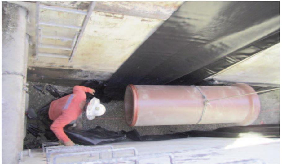
Lowering the new sewer pipe into the trench.
