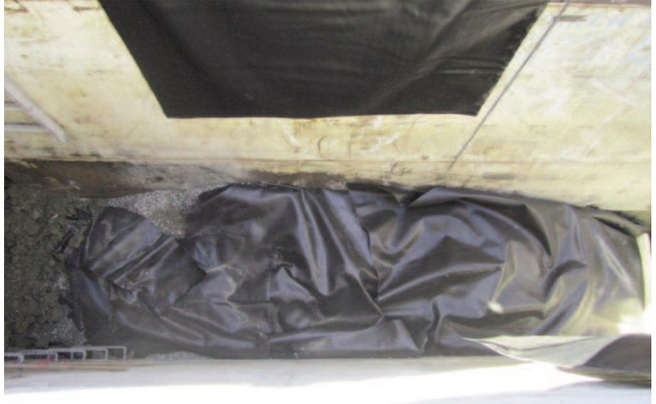
Mirafi® FW700 being cut and then wrapped around the new sewer pipe and the aggregate.
