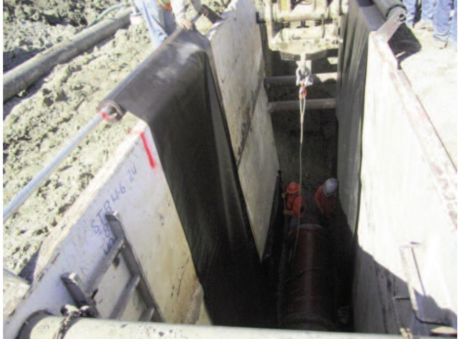
Placing the new sewer pipe upon Mirafi® FW700 and ¾" aggregate.
