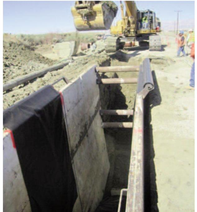
Native soil is used to backfill the trench over Mirafi® FW700.
