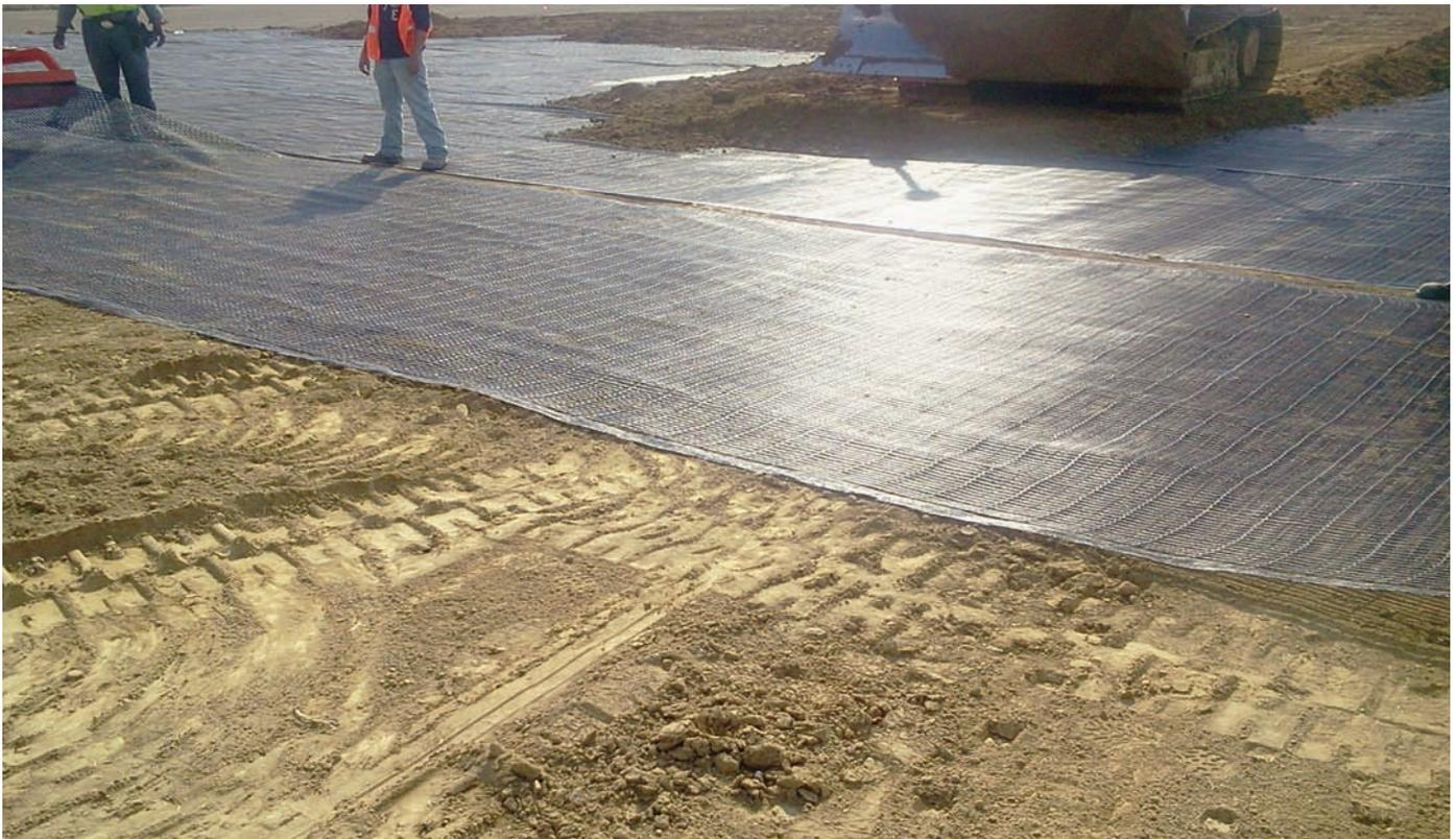
Placement of fill soils on Miragrid® 21XT geogrid.
