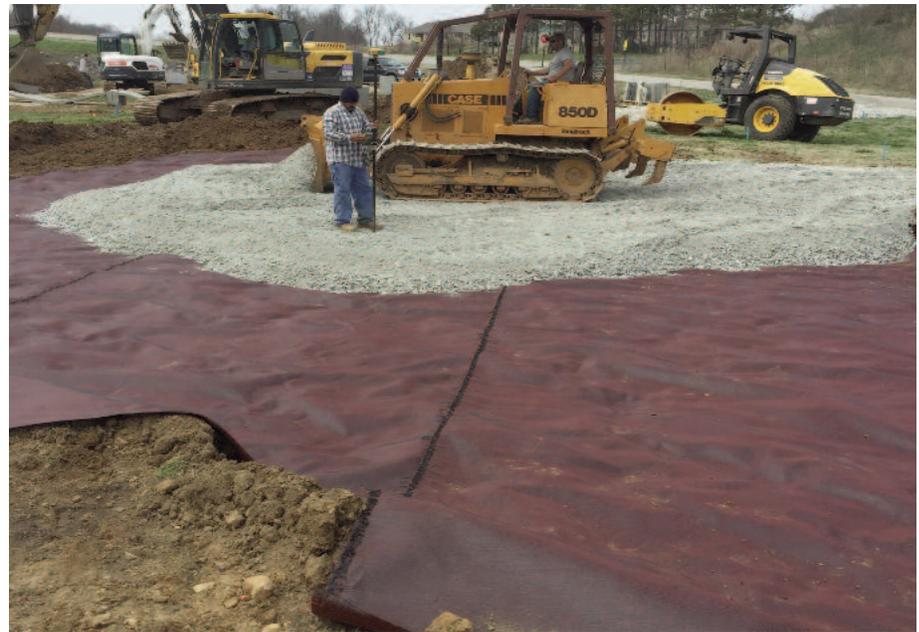
Spreading and compacting the aggregate on top of Mirafi® RS580i.
