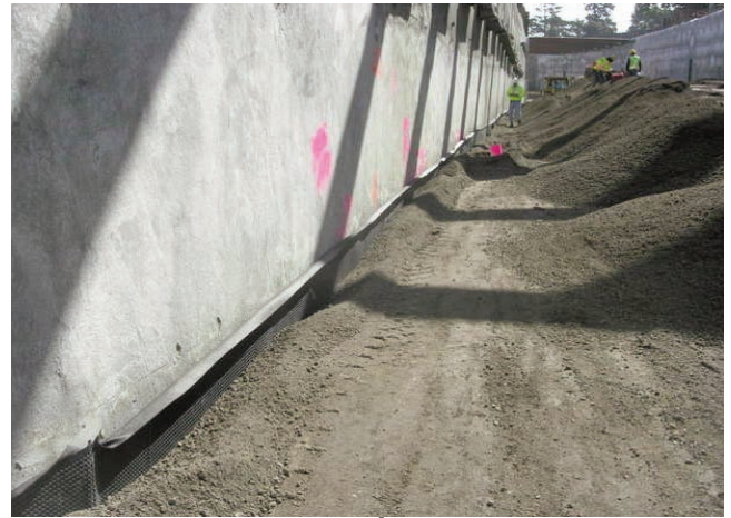
Clean imported fill was placed over Mirafi® RS580i.
