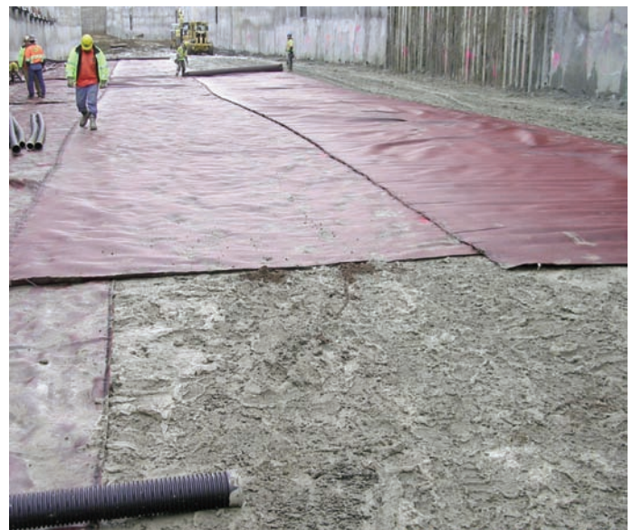
Mirafi® RS580i was laid flat with no wrinkles or folds. A 3' overlap was recommended over the bay mud.
