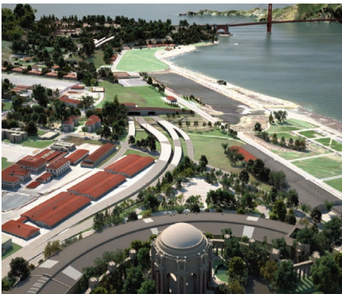
The artist's rendition of the new southern approach to the Golden Gate Bridge that replaces the obsolete structure built in 1936. The contractor encountered soft subgrade while excavating near the Battery Tunnel, center left.
