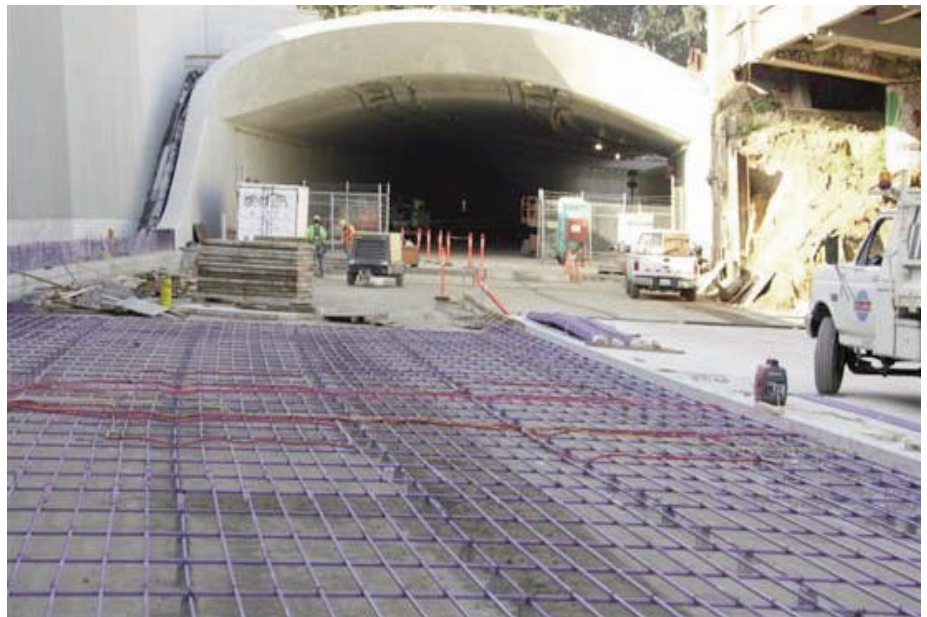
The tunnel entrance nearing completion
