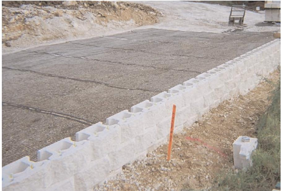
Installed Miragrid® XT Geogrid with Keystone Block.
