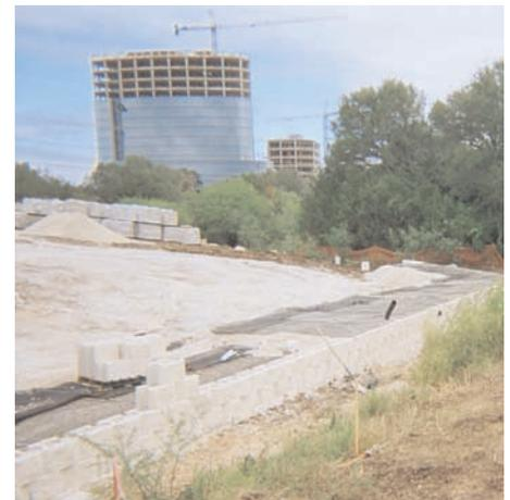
Compaction of aggregate on Miragrid® geogrid.
