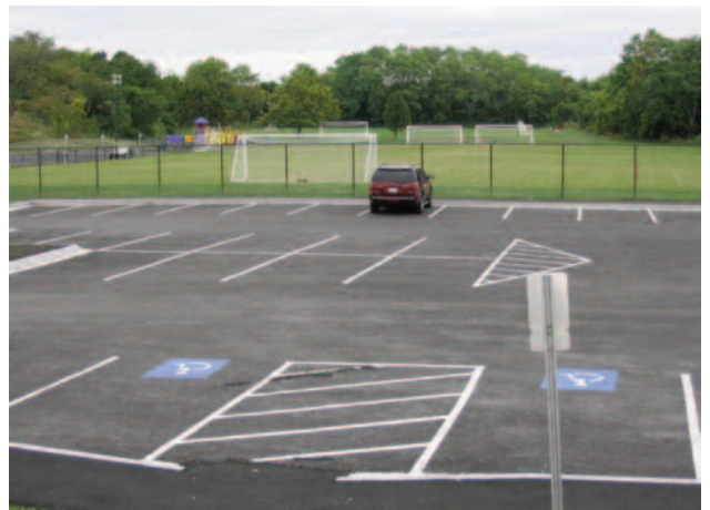
Completed parking lot and soccer fields.
