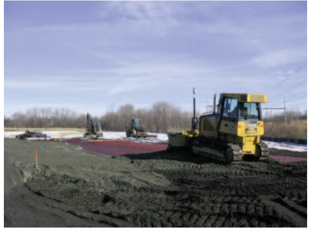
Spreading the structural gravel.
