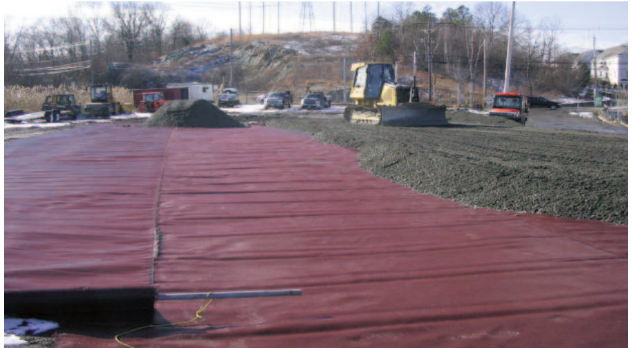
Placement of Mirafi® RS380i geosynthetic with structural gravel.
