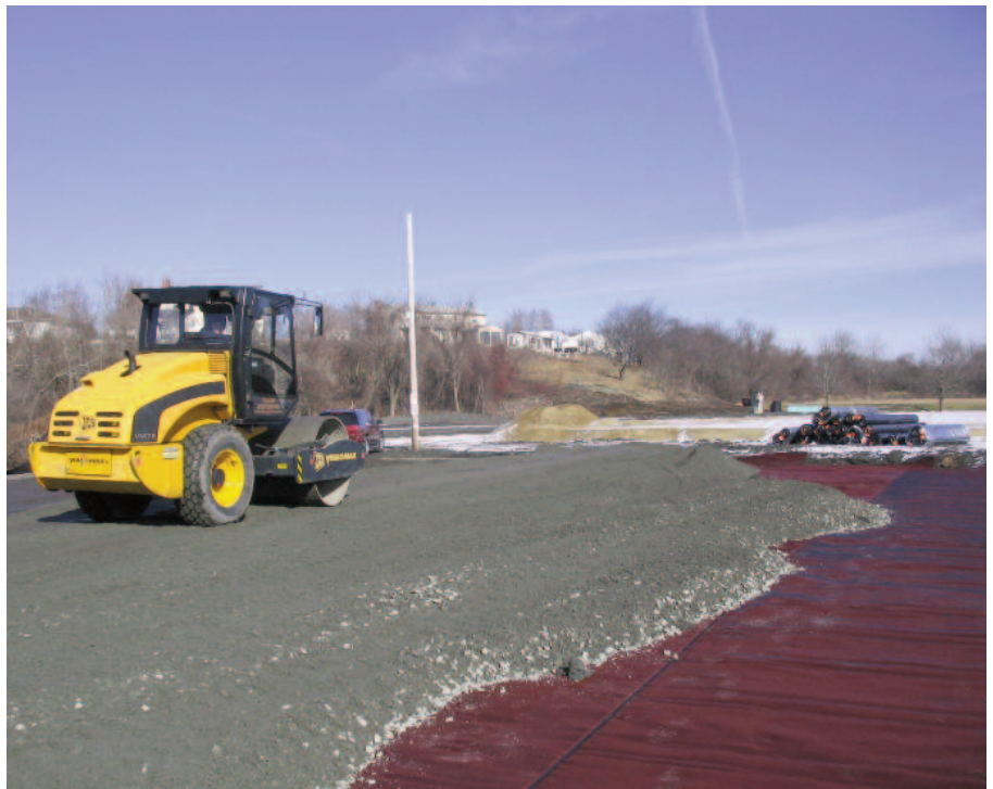
Compacting the structural gravel.
