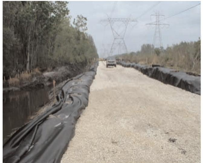
Some areas had to be encapsulated with Mirafi® HP570 and an aggregate in-fill layer.
