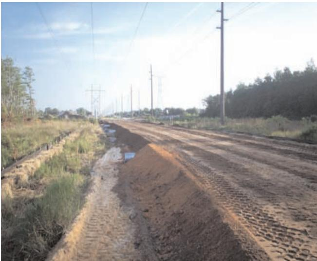
Finished, fully compacted roadway with Mirafi® HP570
