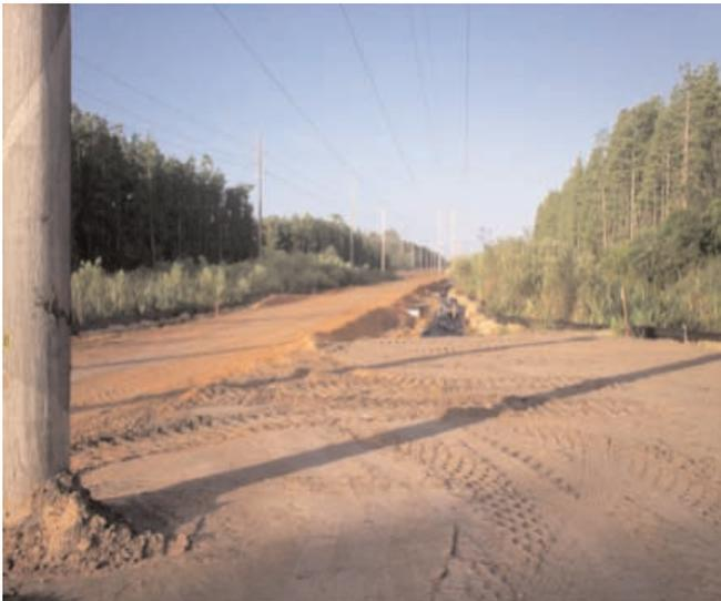
Photo of the pole pads so trucks can work on each pole in time of repairs.
