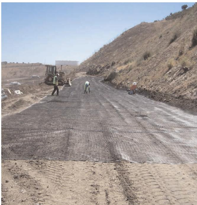
Installing a layer of Miragrid® 8XT.
