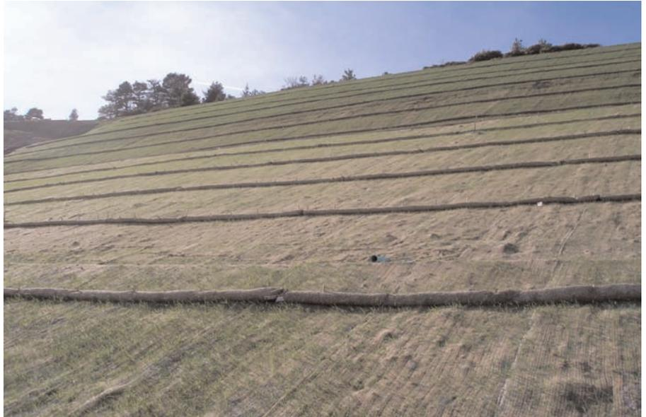
Erosion blankets were used to prevent surface erosion on the manufactured slope.
