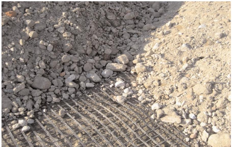
Close-up of recycled concrete base course aggregate placed on Mirafi® BXG11.
