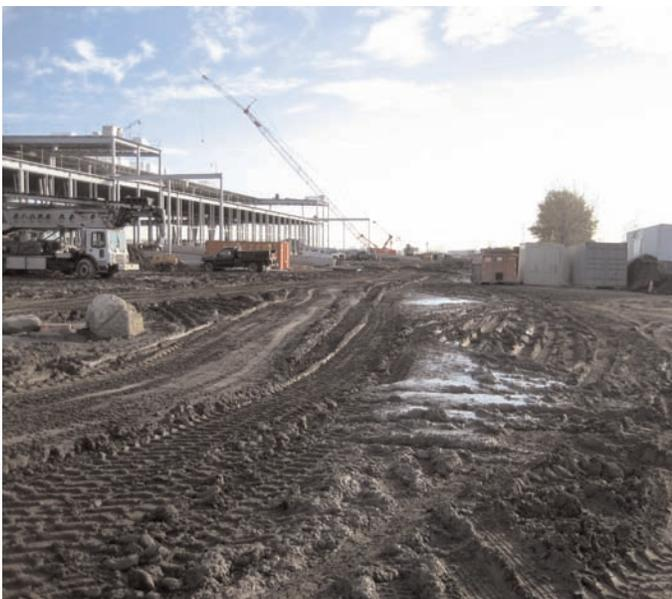
Soft, wet unsuitable on-site soils prior to placement of Mirafi® BXG11 geogrid.
