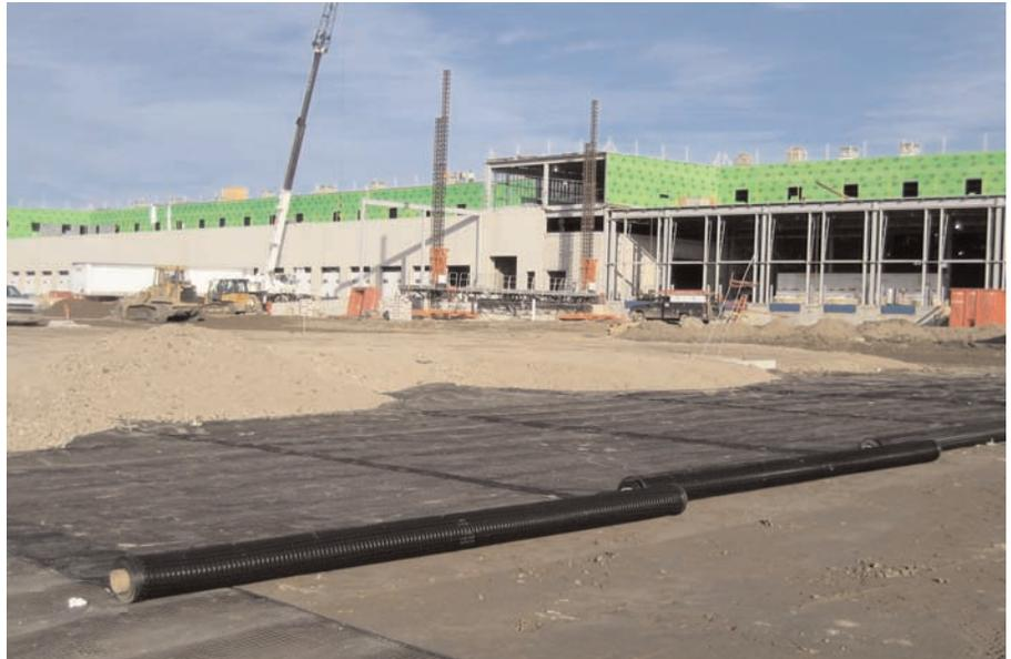
Rolls of Mirafi® BXG11 being deployed over areas of soft subgrade soil.
