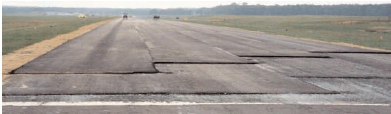
The Person County Airport extended the runway to accommodate larger aircraft. Mirafi® MPV provides a waterproof barrier that extends the pavement life of the overlay.
