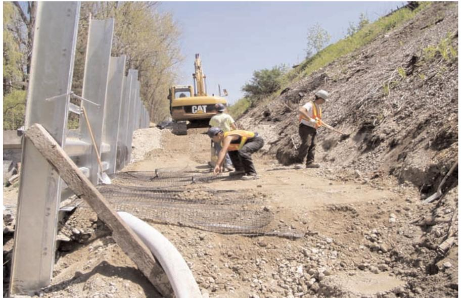
Tensioning of 1m (39in) geogrid wrap back at fascia connector.
