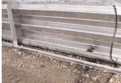
Miragrid®/Bin Wall® connector with 1m (39in) wrap back. Pipe protrusions from wall.
