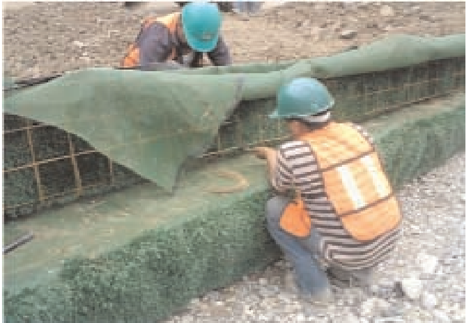
Wire baskets used during wall installation
