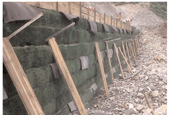
Wood forms used during wall installation
