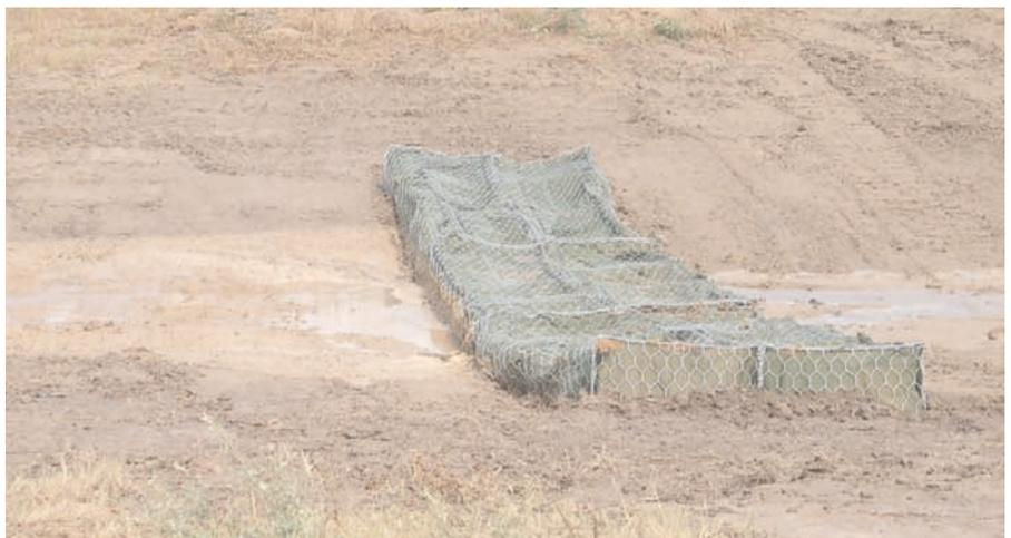
The baskets effectively dam water, allowing sediment to drop out upstream.
