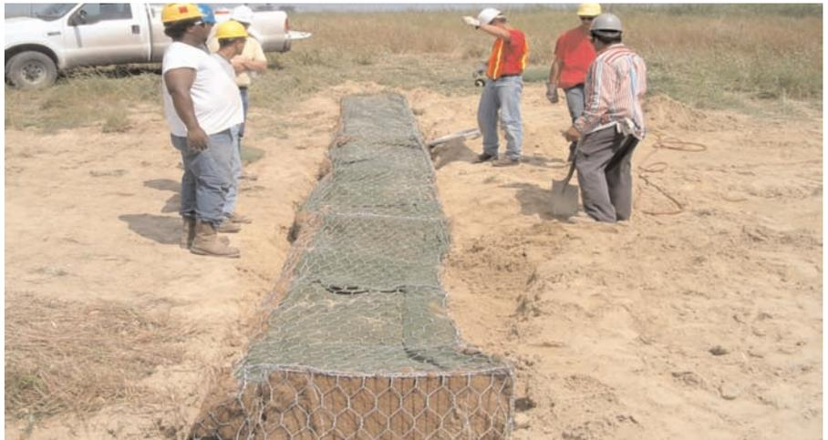
Workers install Miramesh® GR lined gabion baskets in trench across channel.
