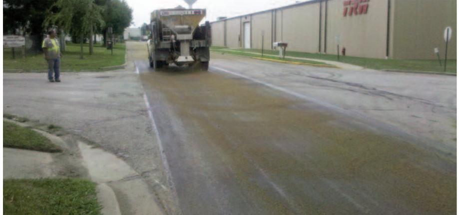
Sanding the Mirafi® MPV500 paving fabric.
