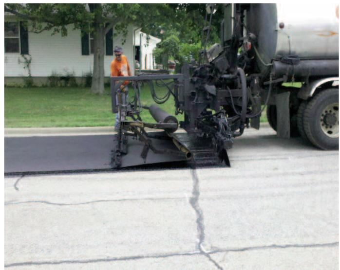
Tack coat and Mirafi® MPV500 being installed.
