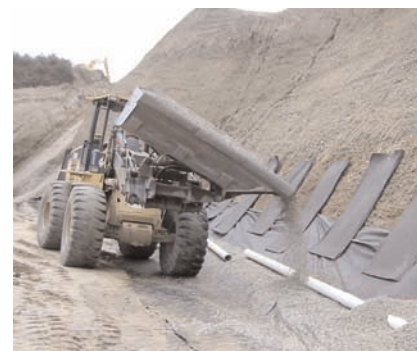
Above: Drain rock being dumped on pipe and Mirafi® 140NC.
