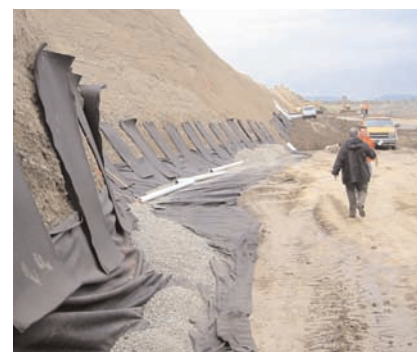
Below: Mirafi® G200N terminating at subdrain system.
