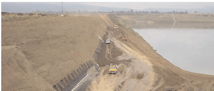
Mirafi® G200N, used as chimney drain, ties into Mirafi® 140NC wrapped subdrain system.
