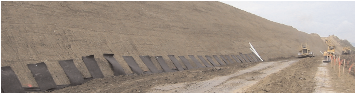
Above: Backfilling of subdrain system. Below: Covering of subdrain system complete.
