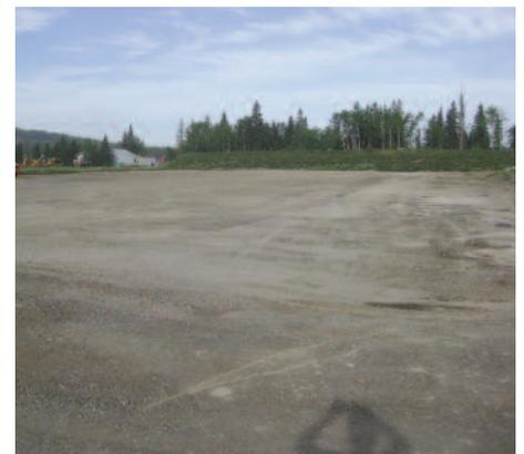
Soft, silty clay material prior to placement of geosynthetic.
