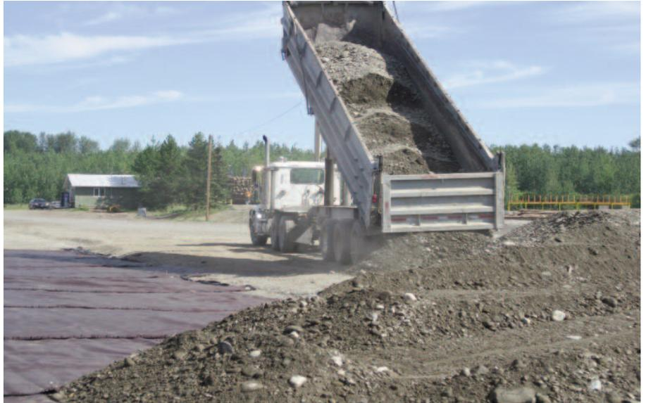
Base material being end dumped on the existing base material.
