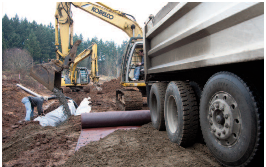
A small amount of aggregate allowed immediate access.
