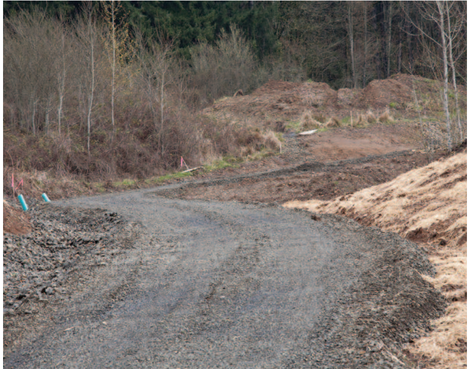
Access road up 12% grade.
