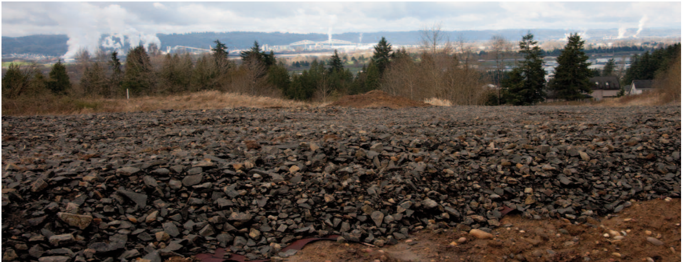
Larger aggregate used over Mirafi® RS380i.
