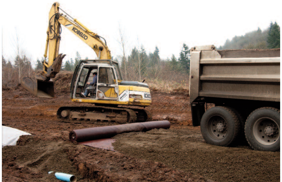
Mirafi® RS380i used for site access.
